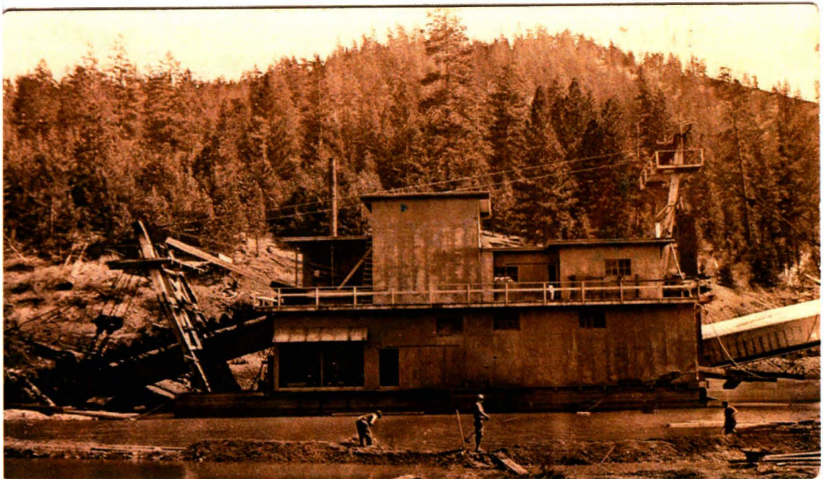
Figure 6. The first and largest chain-bucket dredge to operate in Washington processing gravels on Swauk Creek ca. 1915. Central Washington University Archives, Identifier MS002-06-02.
