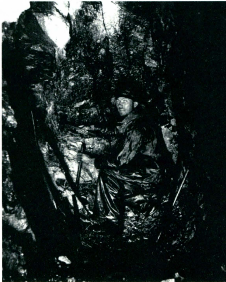
Figure 7. Miner using the single jacking method in the Esther Mine near Gold Creek, Kittitas County, 1898. University of Washington Special Collections, Repository Collection 548.
