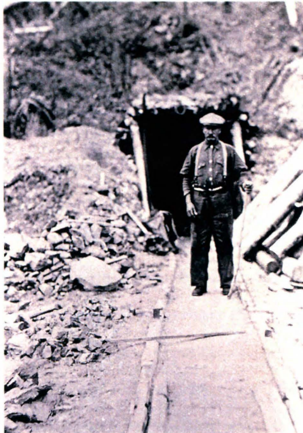
Figure 12. Photograph of a miner in northern Kittitas County at the entrance to an adit. Ore carts were designed to run on tracks or bare earth. Low-grade ore was often stockpiled at the entrance to the mine (left). Ellensburg Public Library Photographs, Identifier MNG-004.
