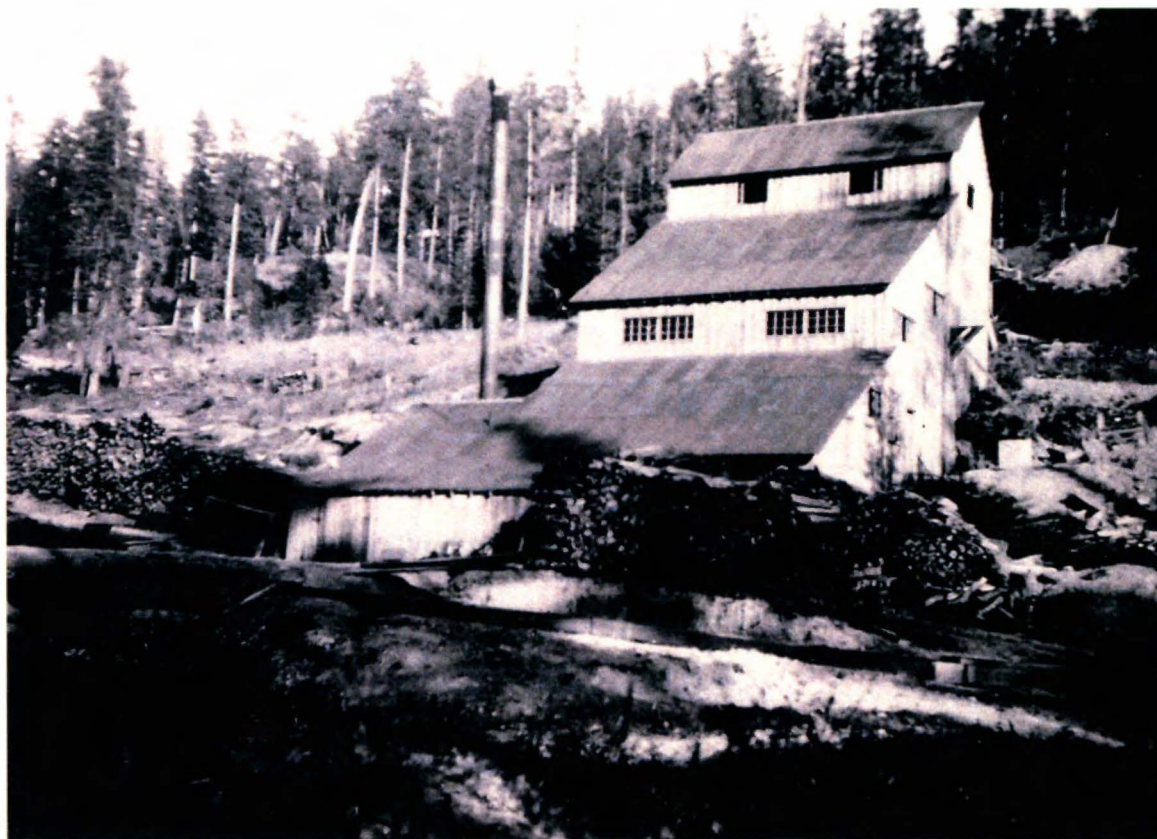
Figure 15. A stamp mill located in the Blewett Mining District. Note how building is built on slope to take advantage of gravity. Ellensburg Public Library Photographs, Identifier MNG-018.
